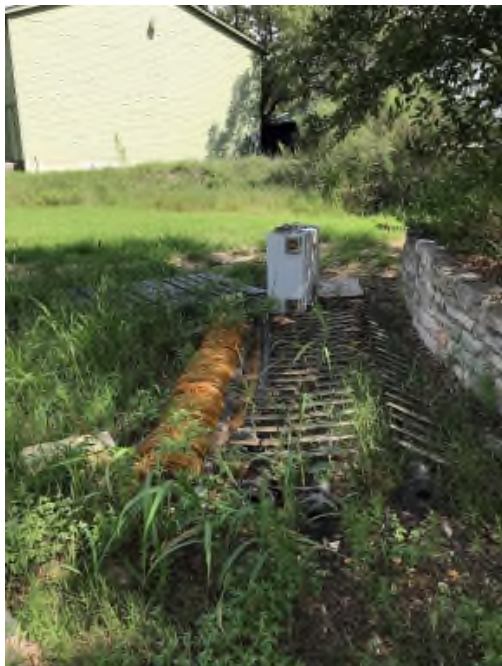
WWTP Site Old Equipment Before
