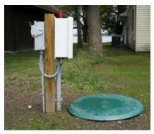
**How do I locate the Grinder Pump on my property**? Your grinder pump station is located between your home and the wastewater main line at the curb. There will be an underground tank that has a cover, similar to the photo to the left, as well as an electrical control panel for the pumping system. Some control panels have been installed inside the garage.
